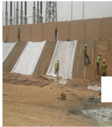
Slope Protection Works
