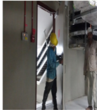
Doors Final Alignment And Installation
